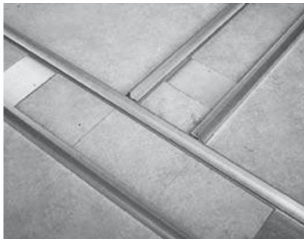
Fix bottom plate assembly to set out on slab with 20mm masonry pins.
