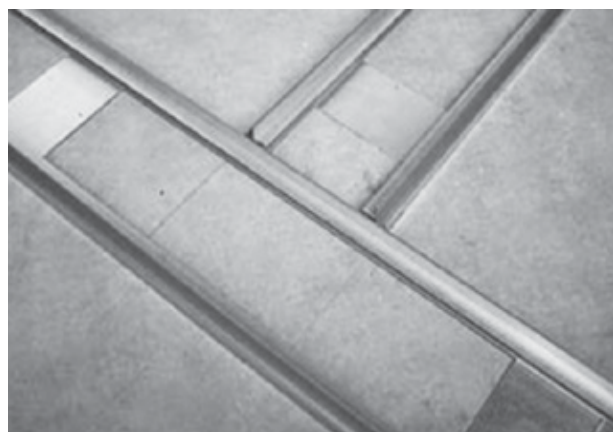
T-Junction Bottom Plate Set-out
