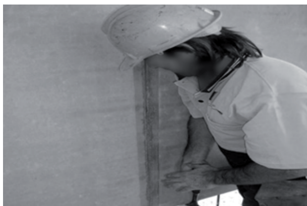
Panel is lifted over starter bars, slid over the Panel Joiners of the fixed panel and then lowered into position.
