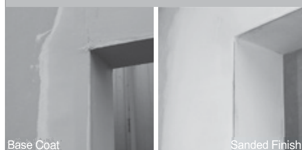
BASE COAT WINDOW / DOOR OPENING FIGURE 5.9
