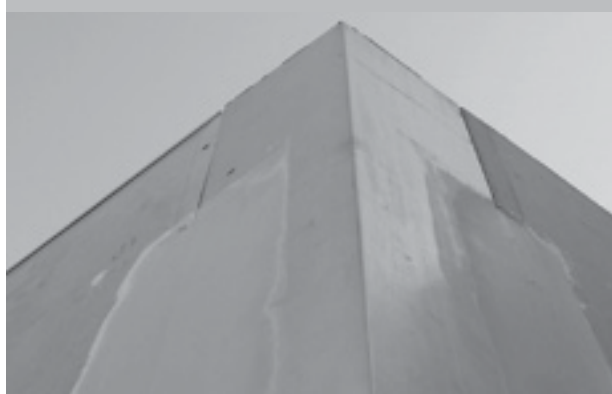
BASE COAT APPLIED TO CORNER CLOSER FIGURE 5.7
